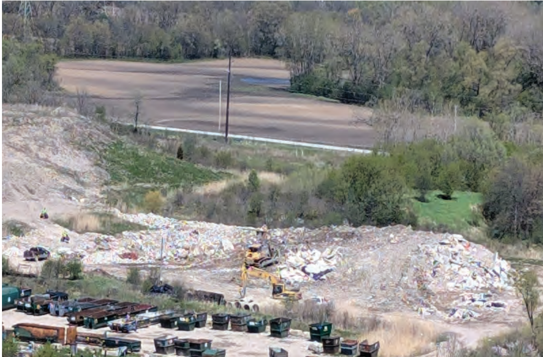
Site making use of concrete stockpile
