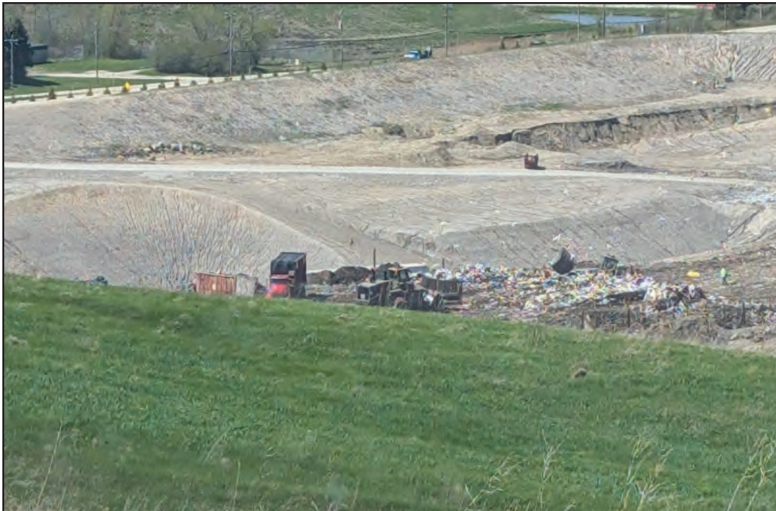
Working face in South end of Phase 4
