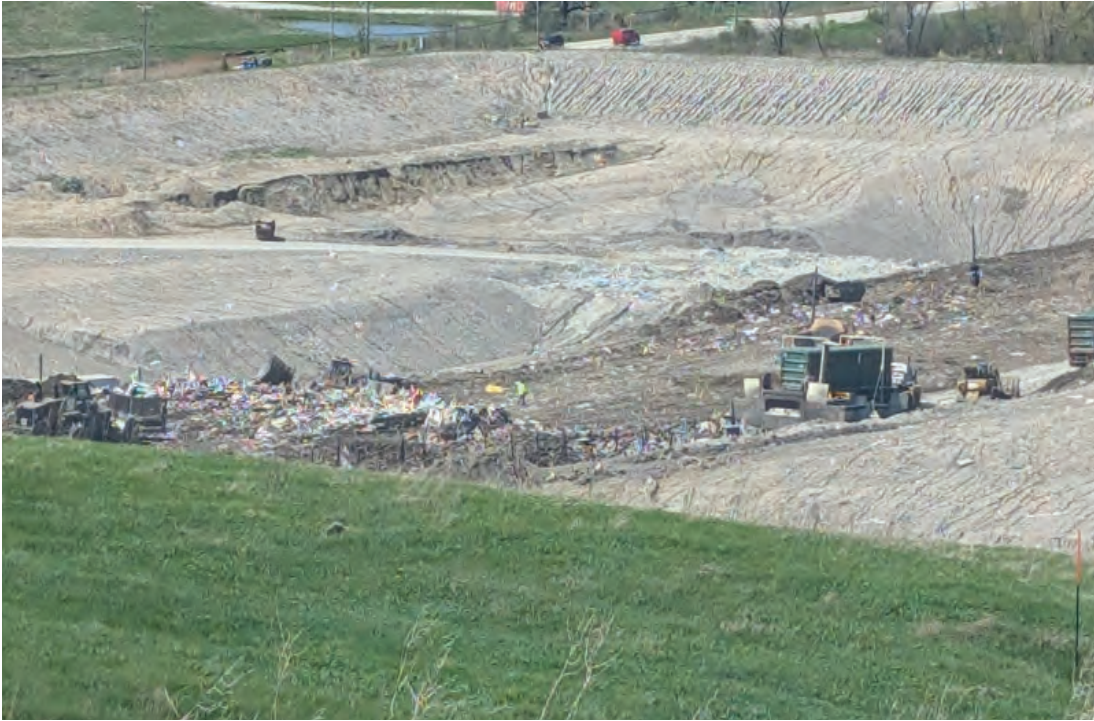
Working face in South end of Phase 4
