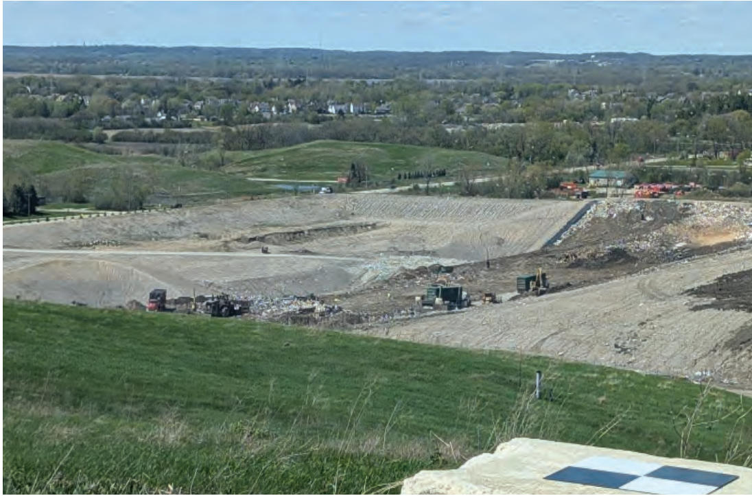
Phase 4 viewed from Southeast
