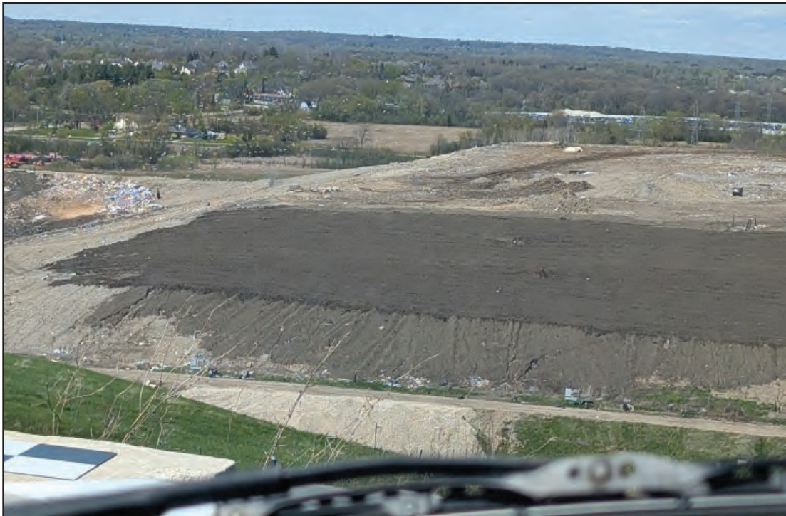
Top soil spread on North slope of North Expansion West
