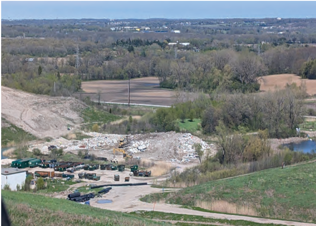
Concrete stockpile being harvested
